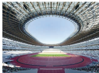
Photos provided by Taisei Corporation
