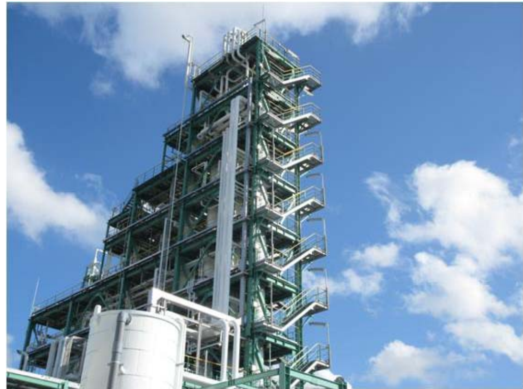
New production facility at the Chiba Plant in Japan
