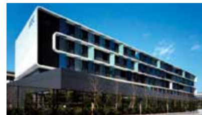
Accommodation facility at the AGC Monozukuri Training Center
