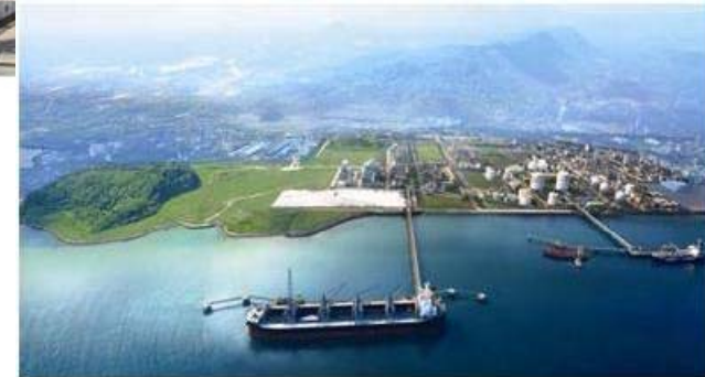
Plant of PT Asahimas Chemical (Indonesia)
