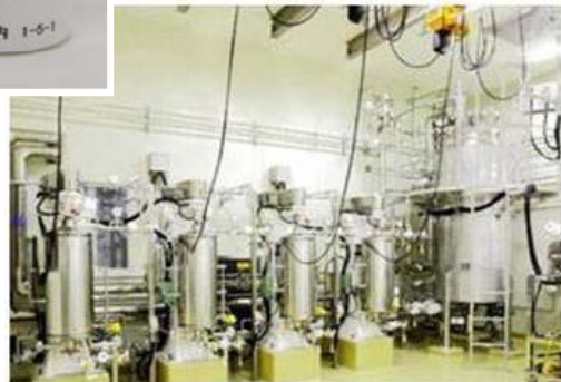
bio-pharmaceutical manufacturing facility
