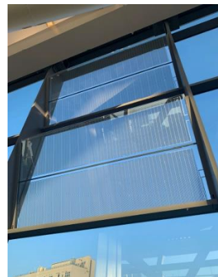
Sunjoule™ SUDARE installed as the station's windows
