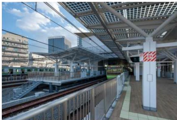
Sunjoule™ adopted for the platform roof
