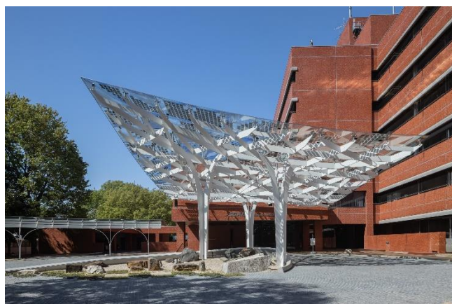
The canopy is sloped to create a welcoming image for visitors.
