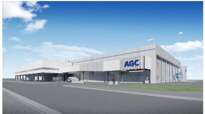
The Motomiya Plant, AGC Electronics' manufacturing base for EUVL mask blanks
