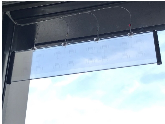
Installed glass antenna
