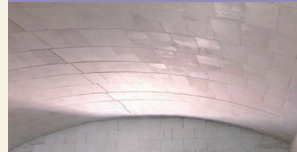
Glass production furnace using fused cast bricks
