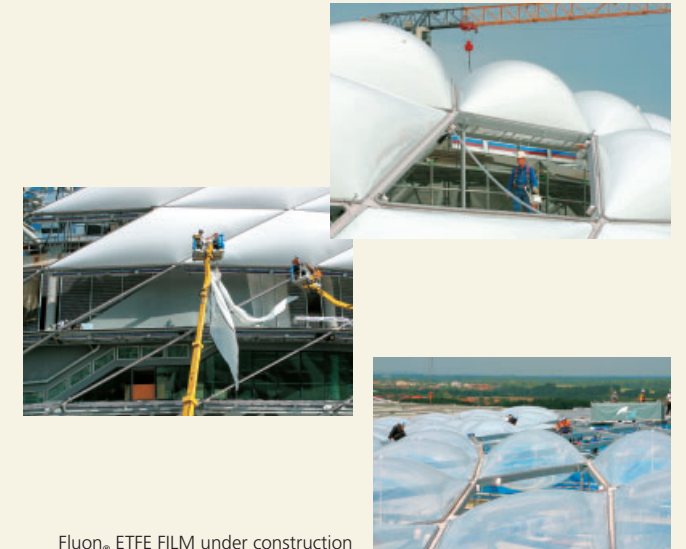
Fluon® ETFE FILM under construction
