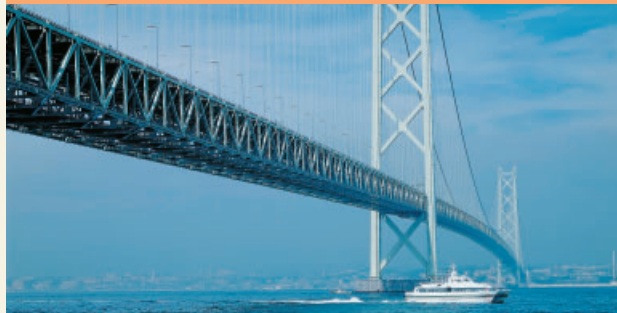
Bridge coated with "Lumiflon," a fluorinated resin for high weather-resistance coatings
