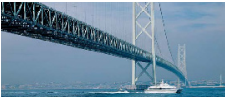
Akashi Kaikyo Bridge painted with long life fluorinated coating (Lumiflon®)
