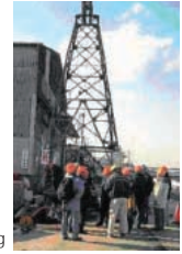
Inspection of soil boring
