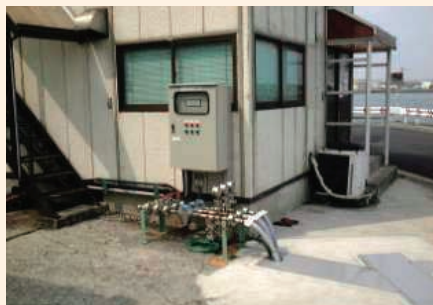
Top: Range of installation of impervious wall and pumping equipment. Aquifer is the sand layer that filters water easily, where groundwater is normally found. Impermeable layer is a clay layer that does not allow water to pass through easily. Left: Pumping equipment for contaminated water, with pumped-out groundwater subjected to purification by means of steam distillation.
