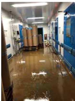
A flooded floor at AGC Pharma Chemicals Europe
