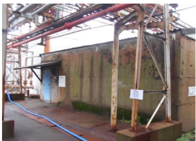
Storage warehouse for PCB waste (Kansai Plant, Amagasaki Factory)
