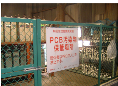
Storage area for PCB waste (YTC)
