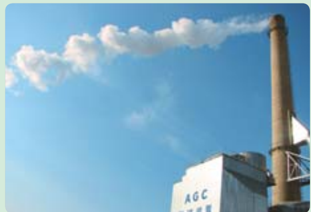
Emitting gas after removing sulfur from it by desulfurization equipment (at AGC Flat Glass (Dalian))
