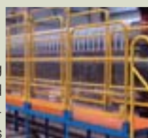
Caustic soda manufacturing facility
