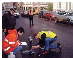
Technicians from Belgian official road laboratory testing the asphalt incorporating the glass
