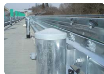
Guardrails for which ETFE caps are used
