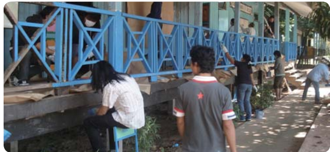
Employees doing repair work for the school
