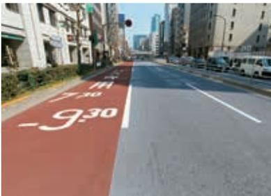
**"Tough Coore™"** ceramic material for heat shielding pavement
