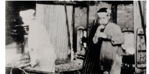
Mass production of flat glass using a Belgian method of producing glass with hand-blown cylinders begins for the first time in Japan. (1909)
