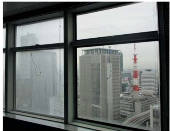
Fig.2 Comparison of condensation between single pane glass and ATTOCH.
