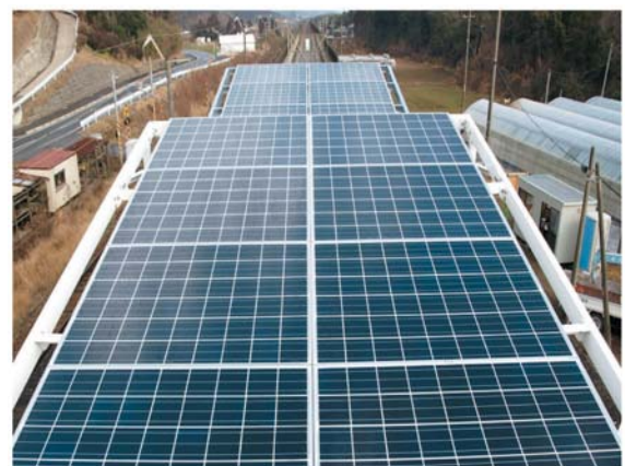
Fig.6 GFRP frame of the solar module for MIYAZAKI solarway.
