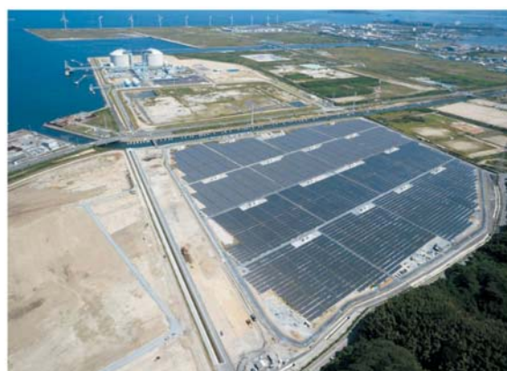
Fig.12 The view of a panorama for “Ene-Seed HIBIKI” photovoltaic power plant.
