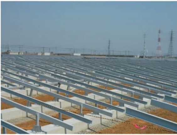
Fig.13 GFRP frame of the solar module by conventional method of construction .
