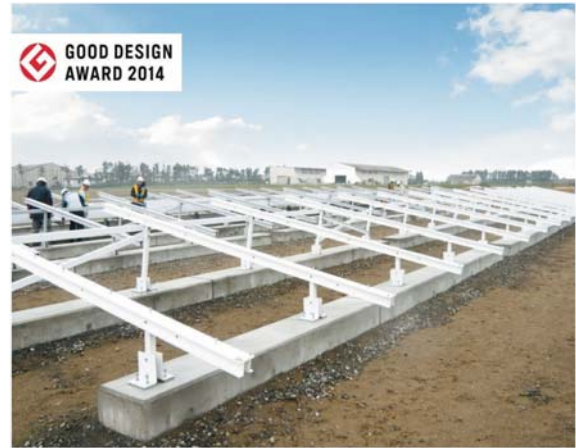
Fig.15 GFRP frame of the solar module by slide construction method.
