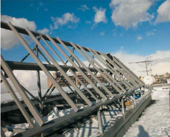
Fig.7 GFRP frame of the solar module for the public facilities in Sapporo.
