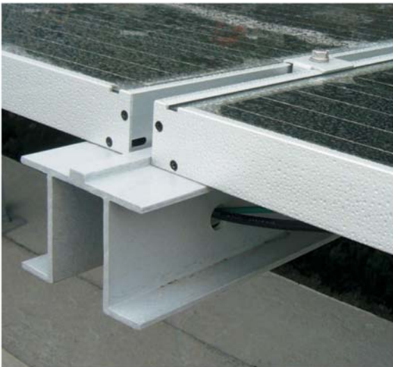
Fig.14 he GFRP-beam similar to the character of “ \pi ”.
