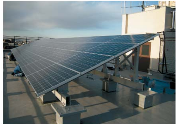
Fig.9 GFRP frame of the solar module for the public facilities in Tokyo.
