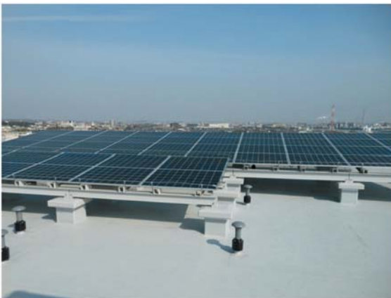
Fig.8 GFRP frame of the solar module for the company's dormitory (AGC).
