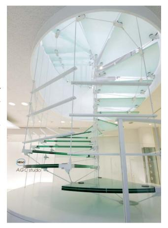
the chemically strengthened specialty glass is used as a building material. With Leoflex, a thin but strong and crack-resistant glass, AGC has created safe, lightweight and transparent staircase rails. Taking advantage of its thinness and flexibility, Leoflex can be installed without any prior bending work. The curved handrails were created simply by bending two sheets of flat glass laminated together.
