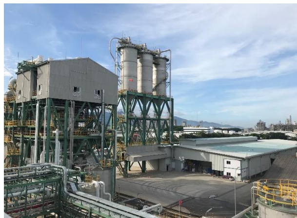
Newly built PVC manufacturing plant
