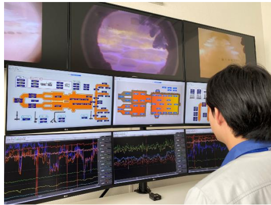
Remote control room for monitoring furnace conditions
