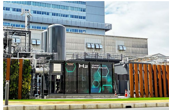
PEM water electrolysis demonstration system (Image provided by Toyota)
