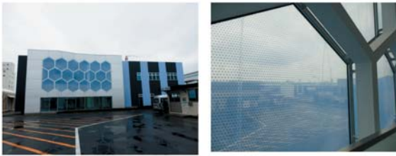
Fig.7 AGC Kashima plant new engineering building and the landscape as seen from the inside
