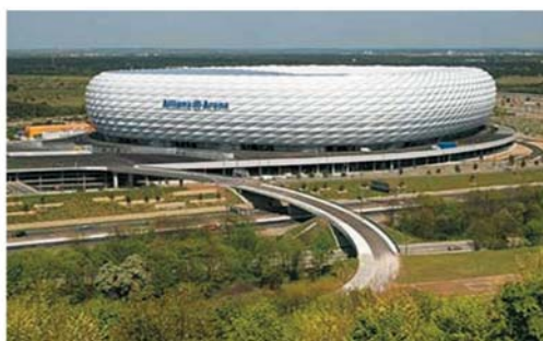
Fig.15 Allianz arena stadium
